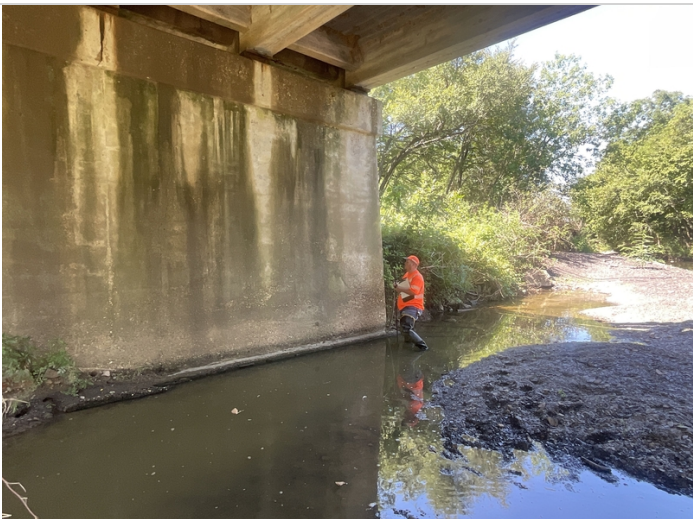
Actual field measurement to document exposed footing elevation.
