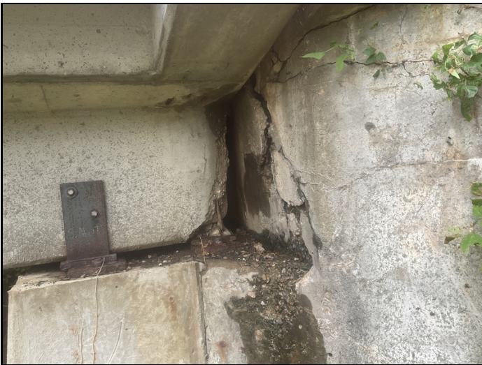
Bent # 1 backwall is leaning towards the channel.
