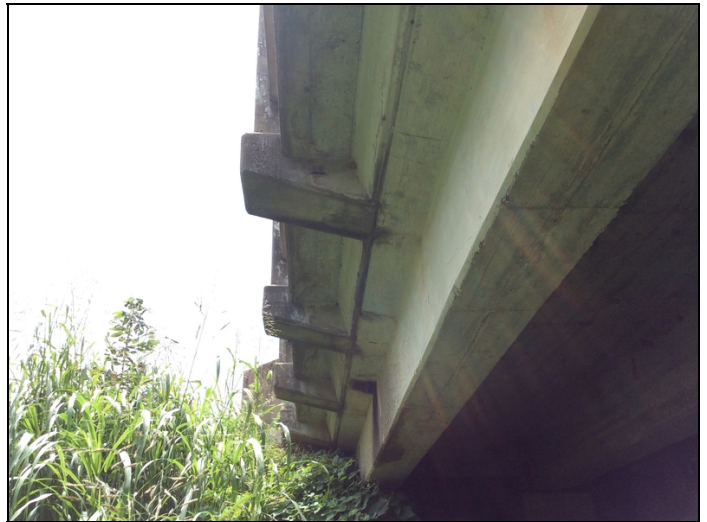
Span # 1 Right Spalling with exposed reinforcing steel in the bridge rails.
