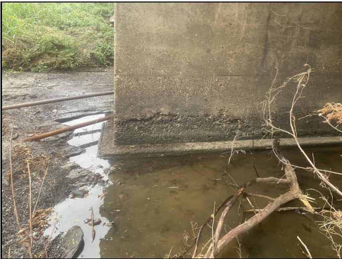
Concrete deterioration at the base of Bent # 3.
