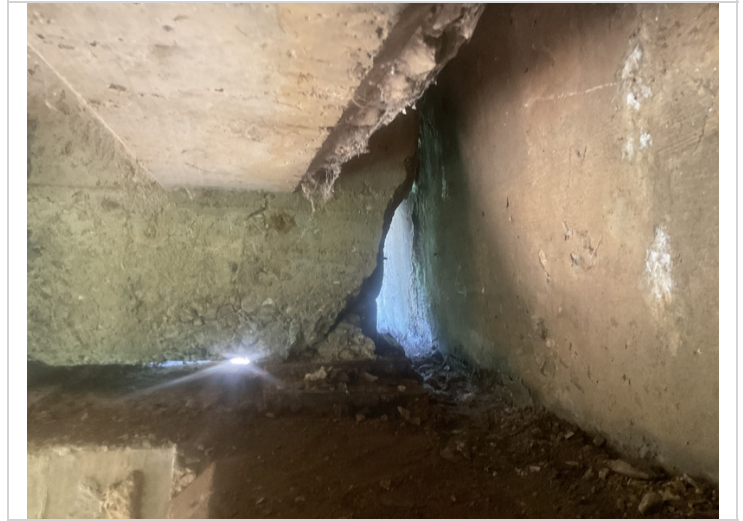
Girder # 5 at Abutment # 1. Spalling with exposed reinforcing steel.
