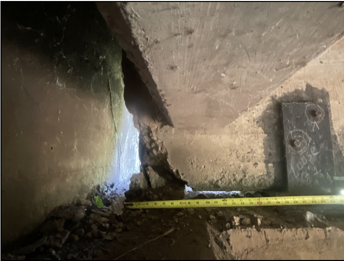
Girder # 1 at Bent # 1. Spalls with exposed reinforcing steel.
