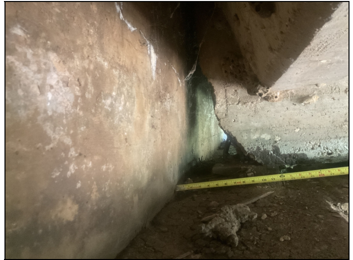
Girder # 2 at Bent # 1. Spalls with exposed reinforcing steel.
