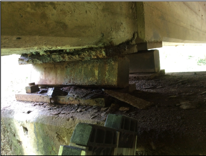
Bent # 2 Girder # 1 Active corrosion with flaking rust in the bearing.
