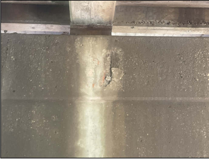
Span # 1 Bent # 2 Spalling with exposed reinforcing steel.
