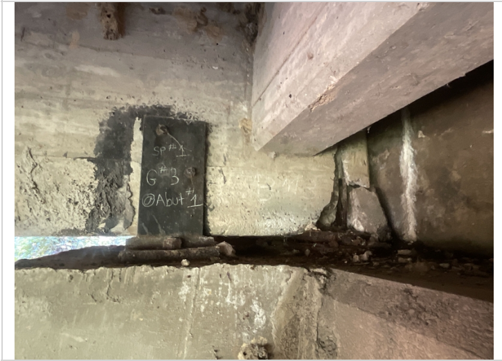
Fixed bearing at Abutment # 1. Girder # 3.
