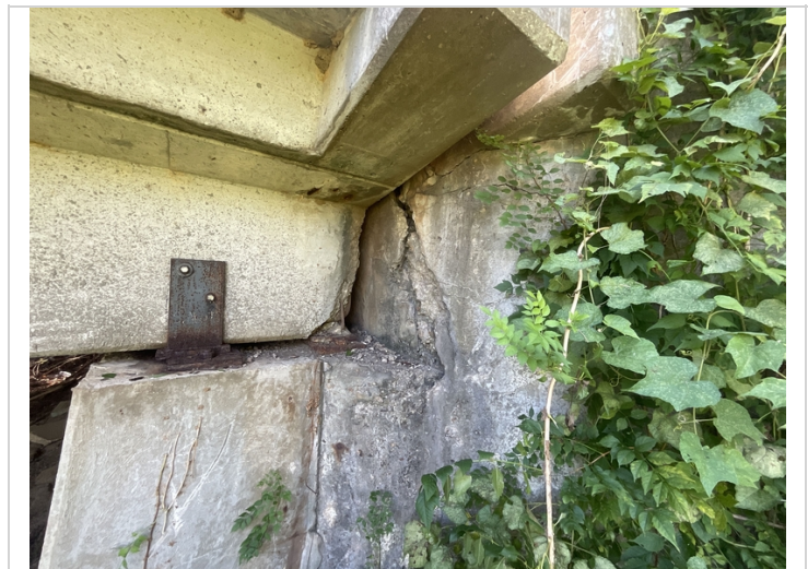
Abutment # 1. Left side. Backwall is fractured and rotated towards the channel.
