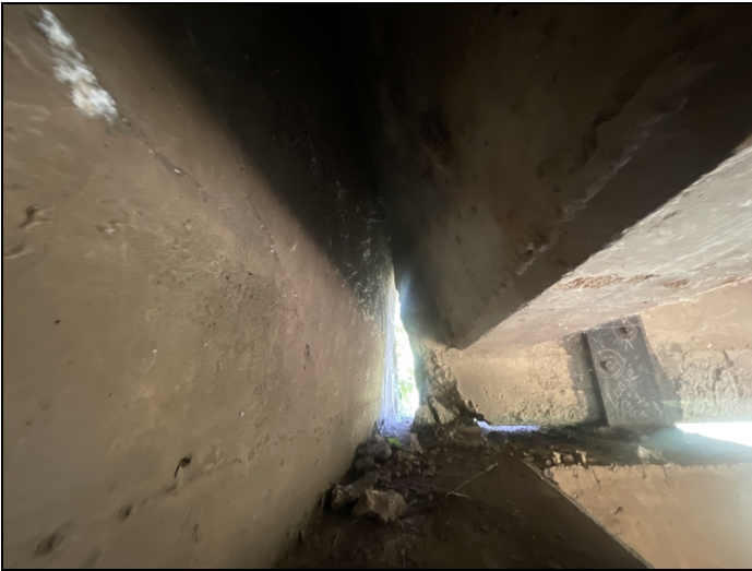
Bent # 1 backwall is leaning towards the channel.
