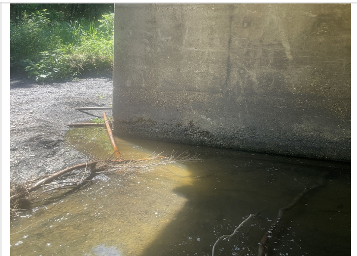
Concrete deterioration at the base of Bent # 3. Ahead face.
