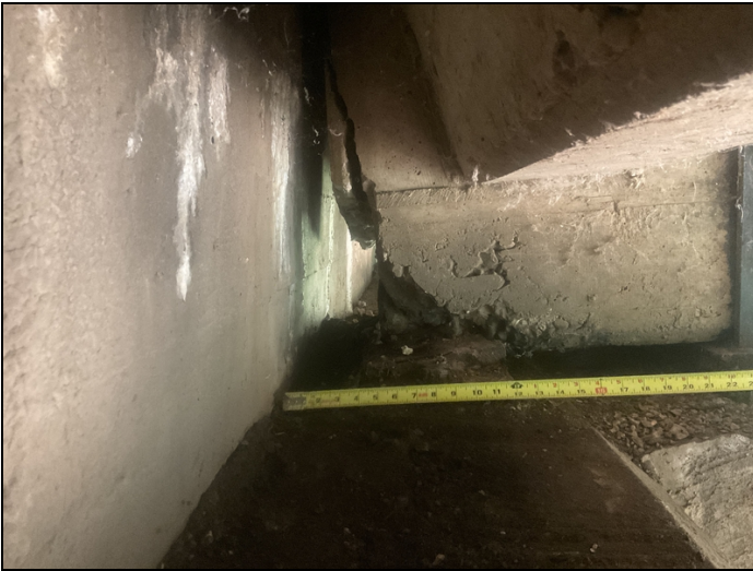
Girder # 1 at Bent # 3. Spalls with exposed reinforcing steel.
