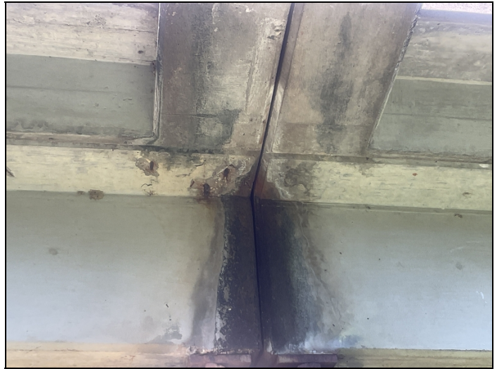
Right overhang of Span # 1 over Bent # 2. Spall with exposed reinforcing steel.
