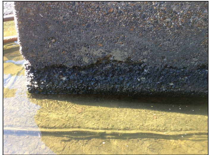
Base of bent # 3 has heavy abrasion with up to 2" of section loss.
