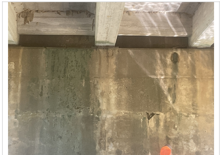
Abutment # 2 cap. Centerline. Spall with exposed reinforcing steel.
