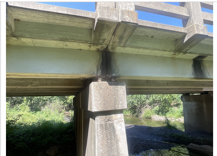
Expansion bearings over Bent # 2. Expanded for Span # 1.
