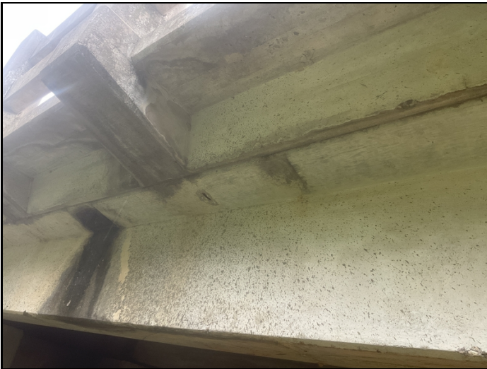
Right overhang of Span # 1. Spall with exposed reinforcing steel.
