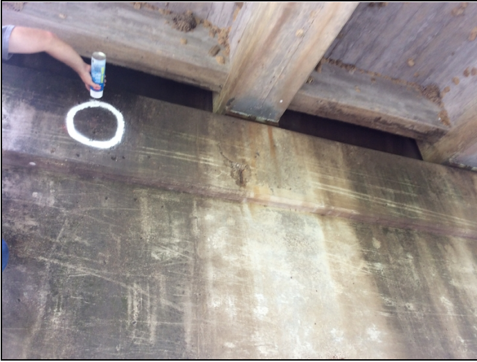
Bent # 3 Span # 3 Spalling with exposed reinforcing steel.
