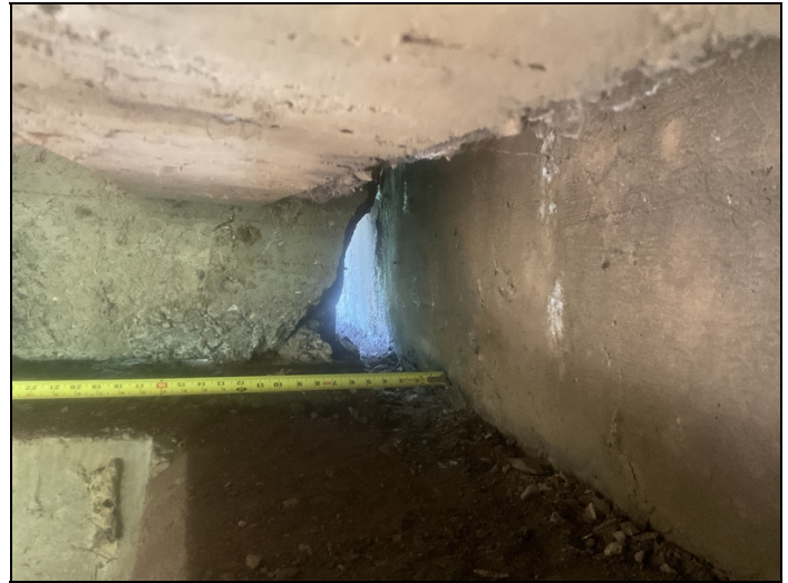
Girder # 1 at Bent # 5. Spalls with exposed reinforcing steel.
