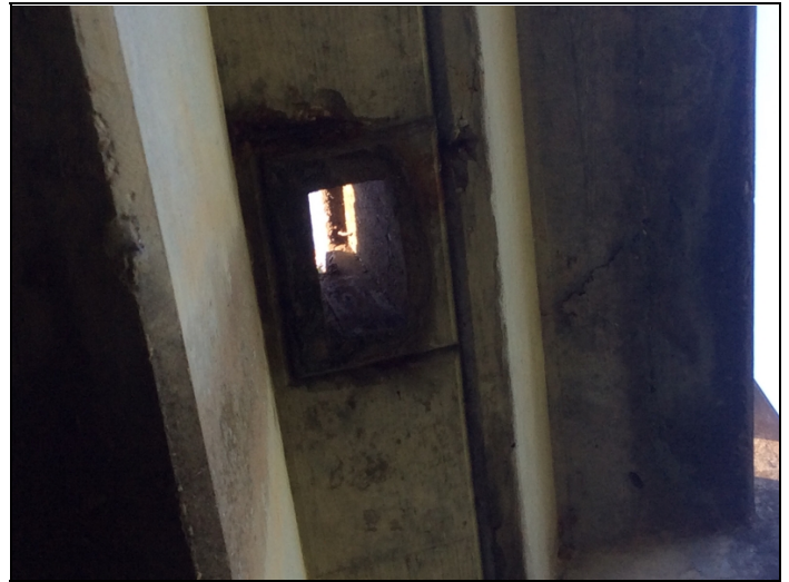
Span # 1, left side-Spalling with exposed reinforcing steel adjacent to deck drain.
