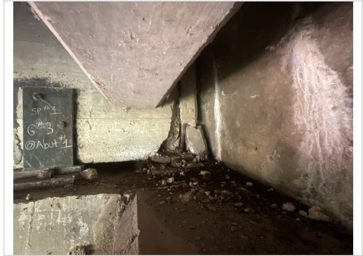
Girder # 3 at Abutment # 1. Spalling with exposed reinforcing steel.
