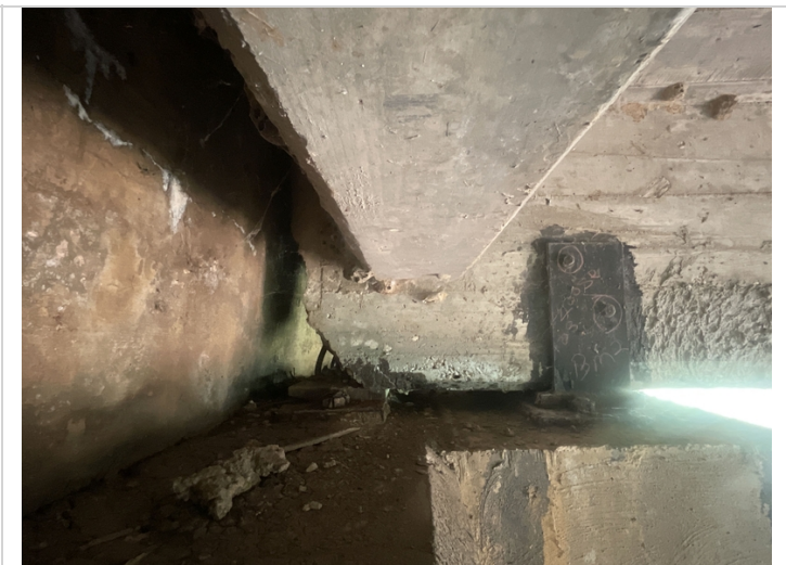
Fixed bearing at Abutment # 1. Girder # 2.
