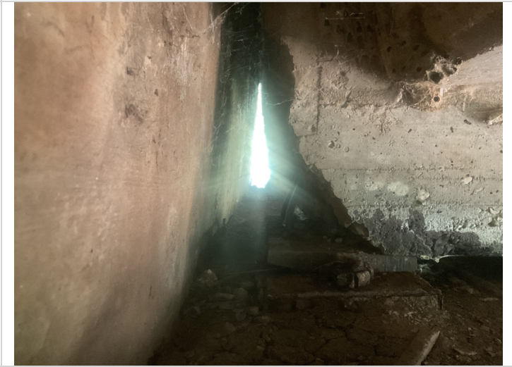
Girder # 2 at Abutment # 1. Spalling with exposed reinforcing steel.
