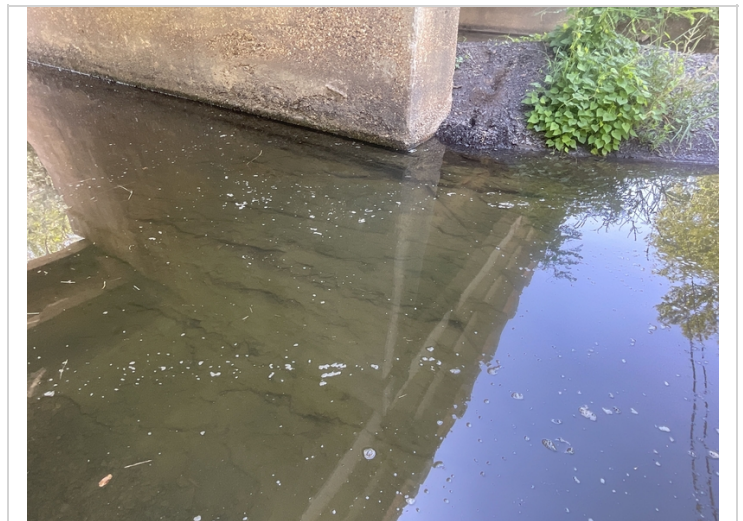
Bent # 3 footing exposed. Solid shale channel.
