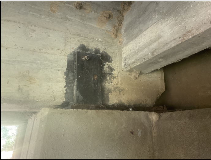
Bent # 1. Girder # 2. Retrofit bearing has fractured and missing bolts.
