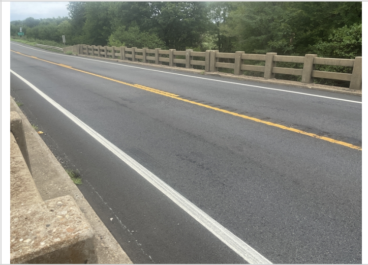
New asphalt wearing surface
