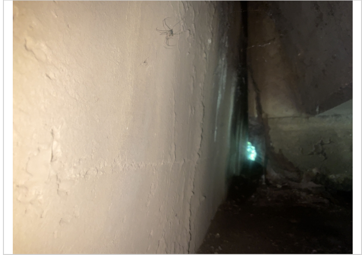
Abutment # 1 backwall makes contact with the ends of the girders at Abutment # 1.
