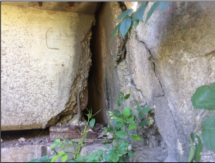
Abutment #1, left side- backwall fractured and rotating.
