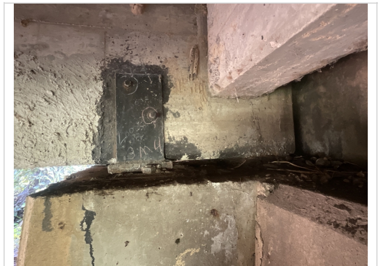
Fixed bearing at Abutment # 1. Girder # 4.
