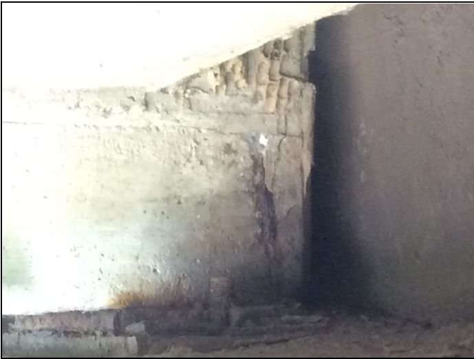
Span # 3, girder # 3 at abutment # 2- Spall with exposed reinforcing steel.
