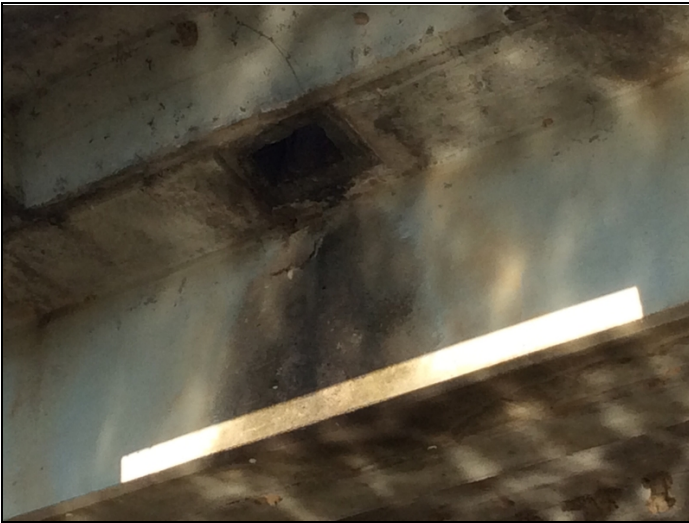
Span # 3, left side of girder # 5- softball sized delaminated area.
