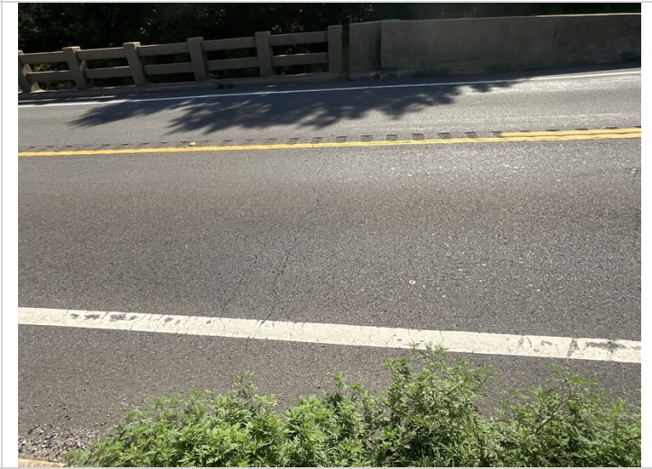
Transverse cracks in the asphalt over Abutment #2 expansion joint.
