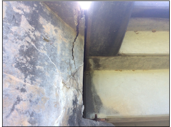
Abutment # 2 backwall, left side- fractured and leaning towards the channel.
