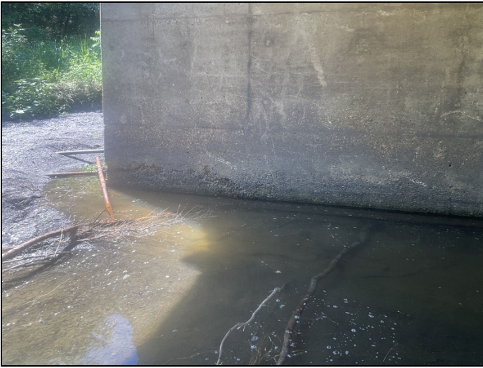
Concrete deterioration at the base of Bent # 3.
