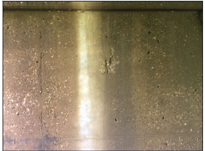
Span # 1 Bent # 2 Spalling with exposed reinforcing steel.
