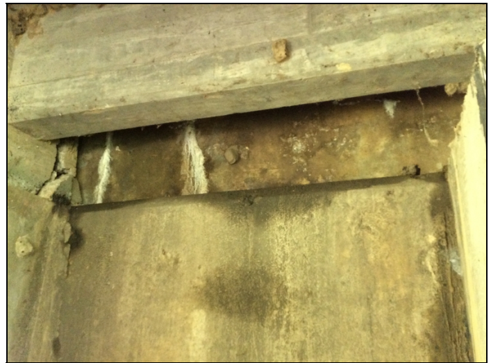
Bent # 1 Back wall cracking. With efflorescence.
