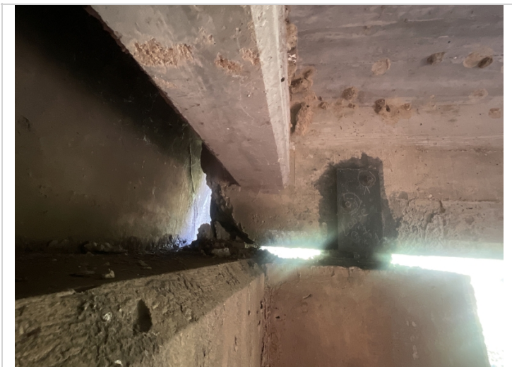
Girder # 1 at Abutment # 1. Spalling with exposed reinforcing steel.
