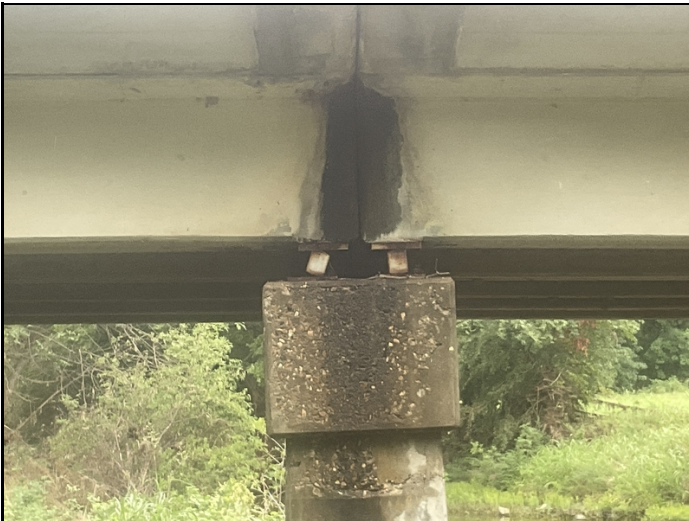
Span # 1, Bent # 2 bearing leaning. Girder # 5. No apparent change since the last inspection.
