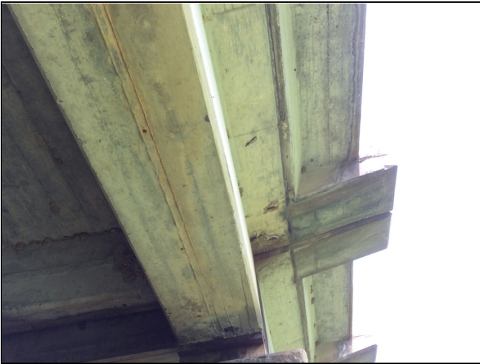
Span # 1 Right Spalling with exposed reinforcing steel.
