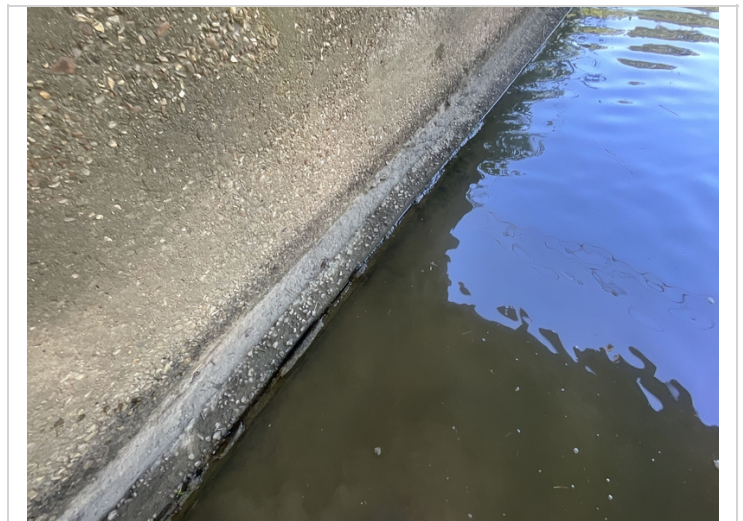
Bent # 2 footing is exposed on the ahead face of the bent.
