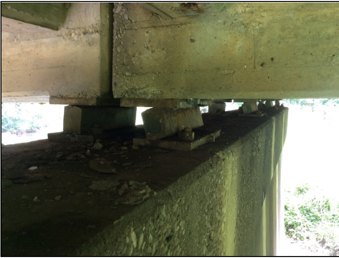
Bent # 2 Span # 1 Bearing movement.
