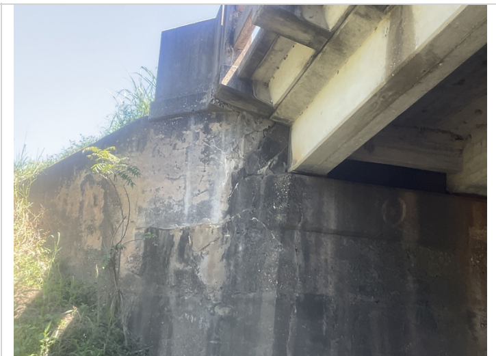
Abutment # 2 - There are delaminated areas and map cracking in the exterior edges of the back walls adjacent to the wing wall connection.
