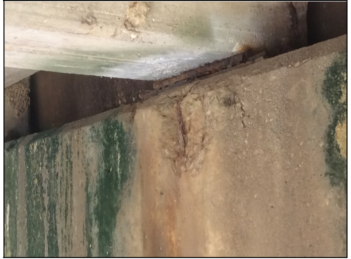
Abutment # 2 spall with exposed reinforcing steel.
